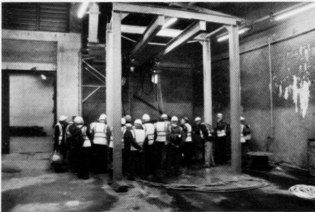
The Sub Brit visitors crowd round for a good view (and not so good smell) of the pump shaft at the storm water storage site. Photo Dom Jackson
